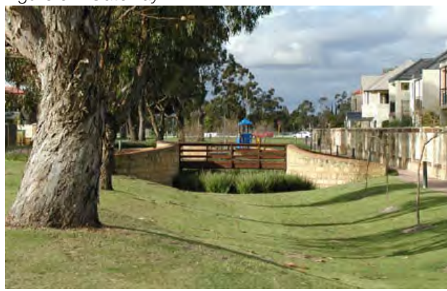
Figure 56. Footpath crossing swale
