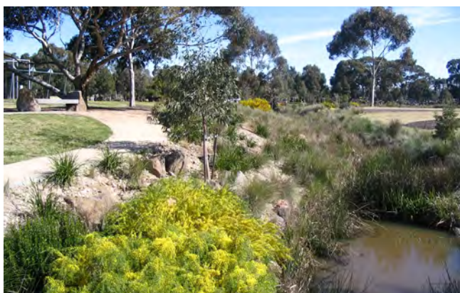
Figure 40. Vegetated swale
