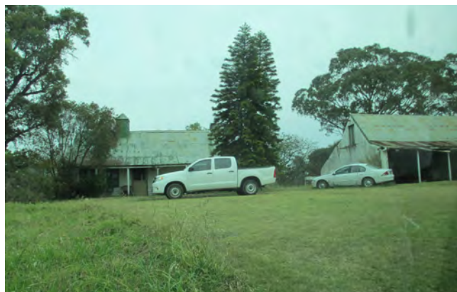
Figure 31. Existing Varroville outbuildings
